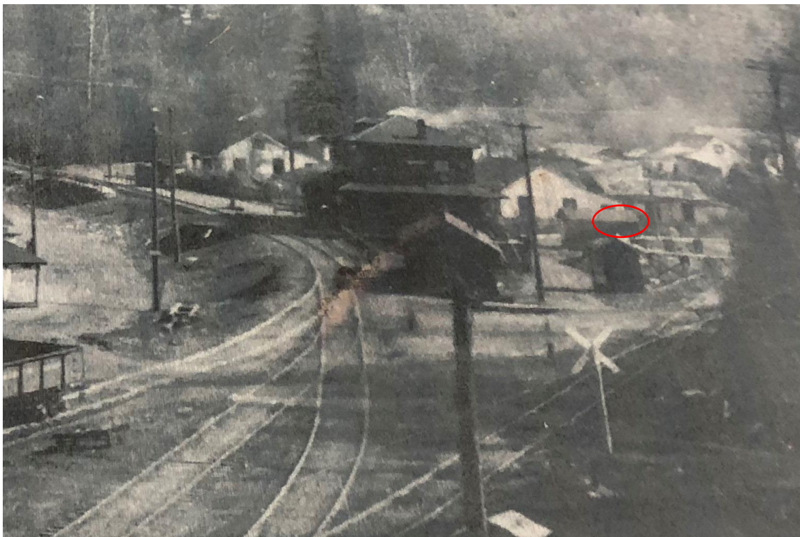
Figure 19. Overview of main railroad grade, rail depot, and turntable area. Location of TU-4 at the end of the turntable spur. Facing northeast. Dated 1927. Courtesy of Foothills Historical Society.
