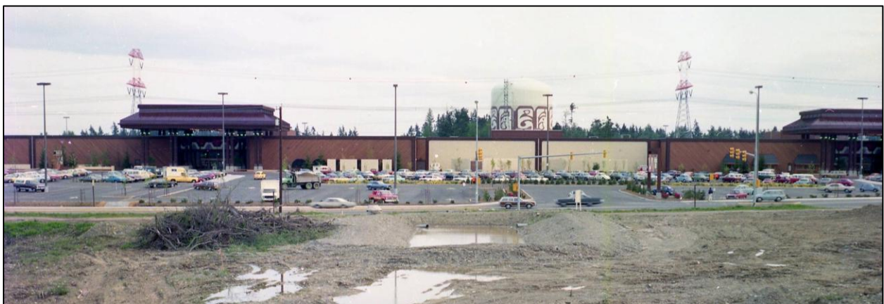
Figure 32. North elevation of SeaTac Mall, view facing south, 1975 (HSFW).
