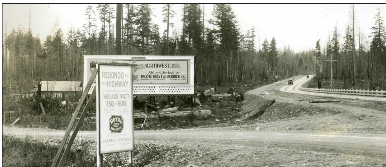
Figure 14. US 99 Pacific Highway looking north with east half paved and west half graded for future pavement, ca. 1929 (Washington State Digital Archives, Ref# AR-28001001-ph000201).
