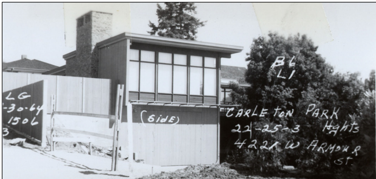
4221 West Armour Street, west elevation, view facing southeast (WA State Archives, July 30, 1964).
