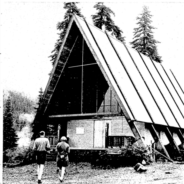
The Chapel of St. Bernard is of sturdy construction to withstand the heavy weight of Cascade Mountain snows. The steel support beams are mounted on huge, concrete anchors.
